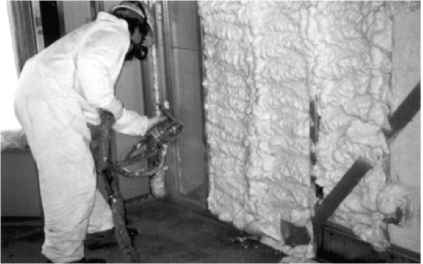
Figure 10.1 Spray application of Icynene. ( Icynene )
